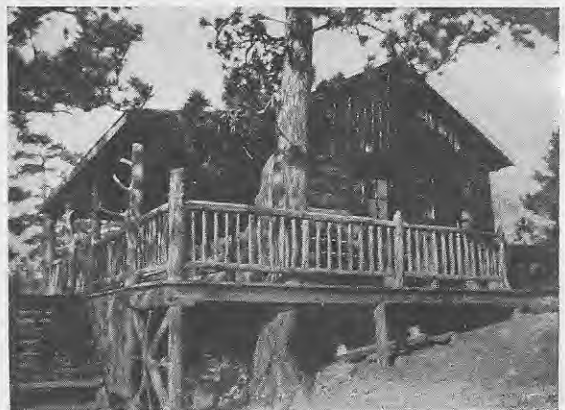
A Few of the Many Cabins Built at Redfeather Lakes
