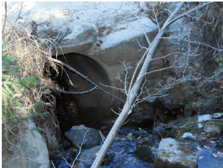
This culvert is about two miles up the Deadman road.
