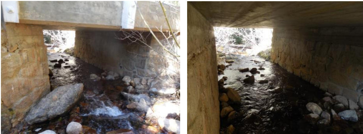
Stone bridge under Deadman Road at Killpecker Creek
