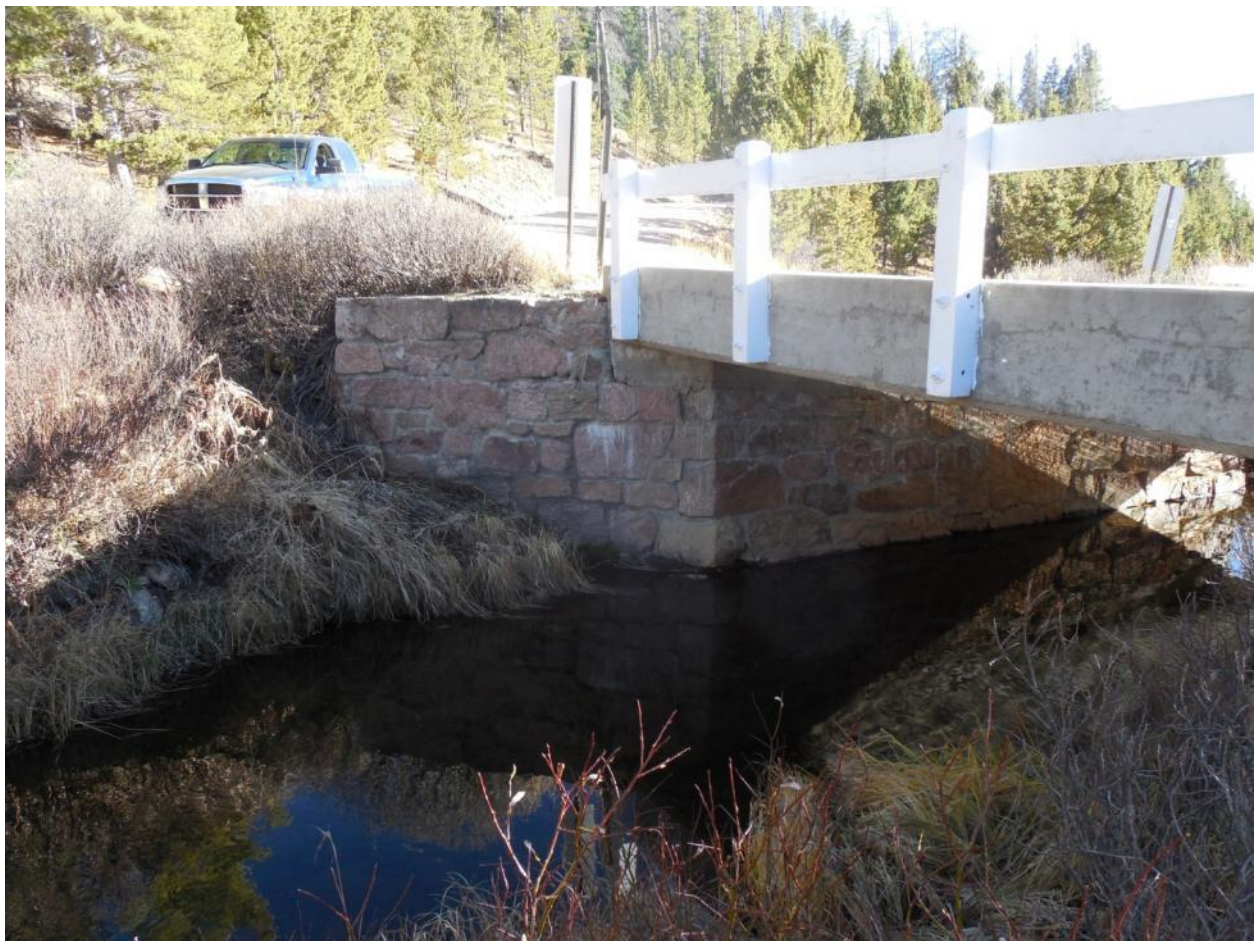
Bridge over Sand Creek on Deadman Road
