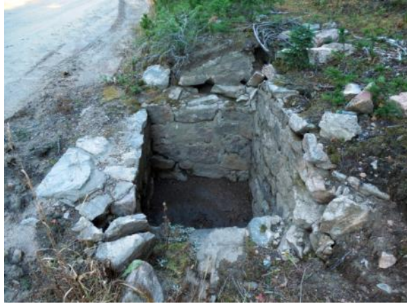
Damaged catch-basin just west of the North Fork Poudre campground.
