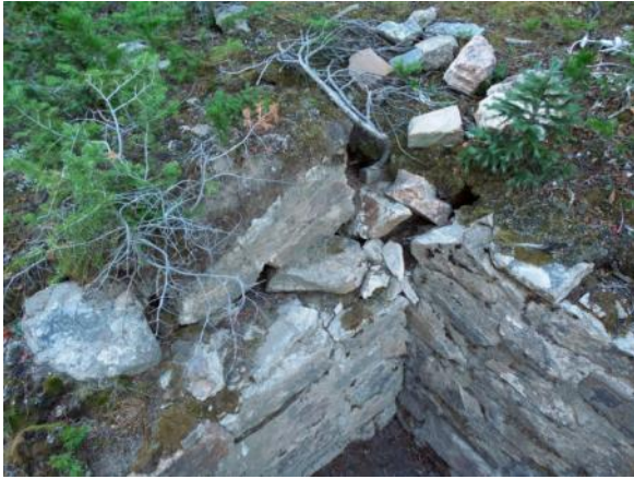
Damaged catch-basin just west of the North Fork Poudre campground.
