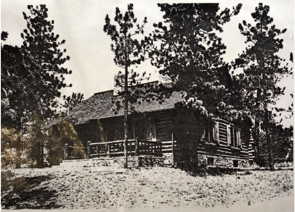
Jul 5, 1949 Ass't Ranger's Residence, Redfeather Ranger Station
