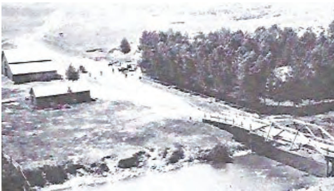
Aerial View of Livermore Hotel
